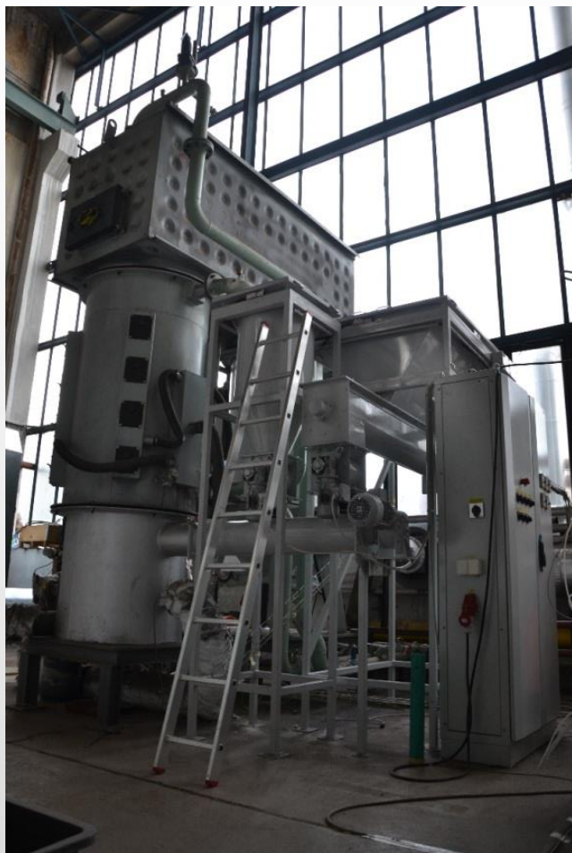
Fluidized bed boiler - 500 kW – oxy fuel combustion (CTU)
