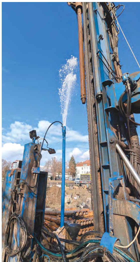
Cleaning of drilling fluid in hydrogeological well LTH-1. This well will be used as hydrogeological monitoring borehole in the BTES field at the Litoměřice locality. Photo by J. Holeček.
