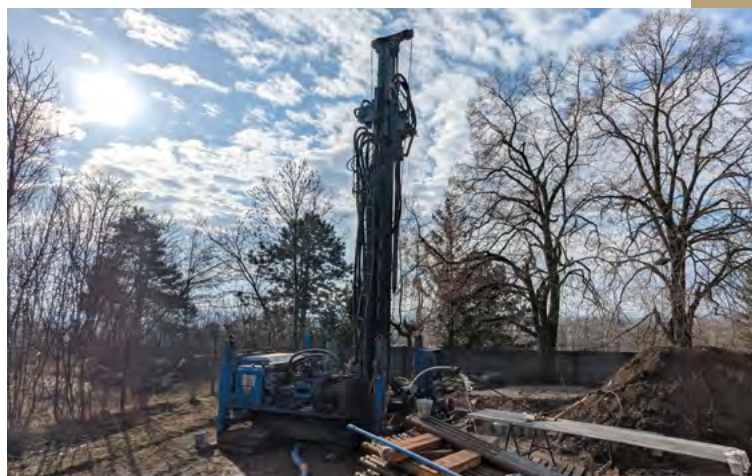
Cleaning of drilling fluid in hydrogeological well LTH-1. Photo by J. Holeček.
