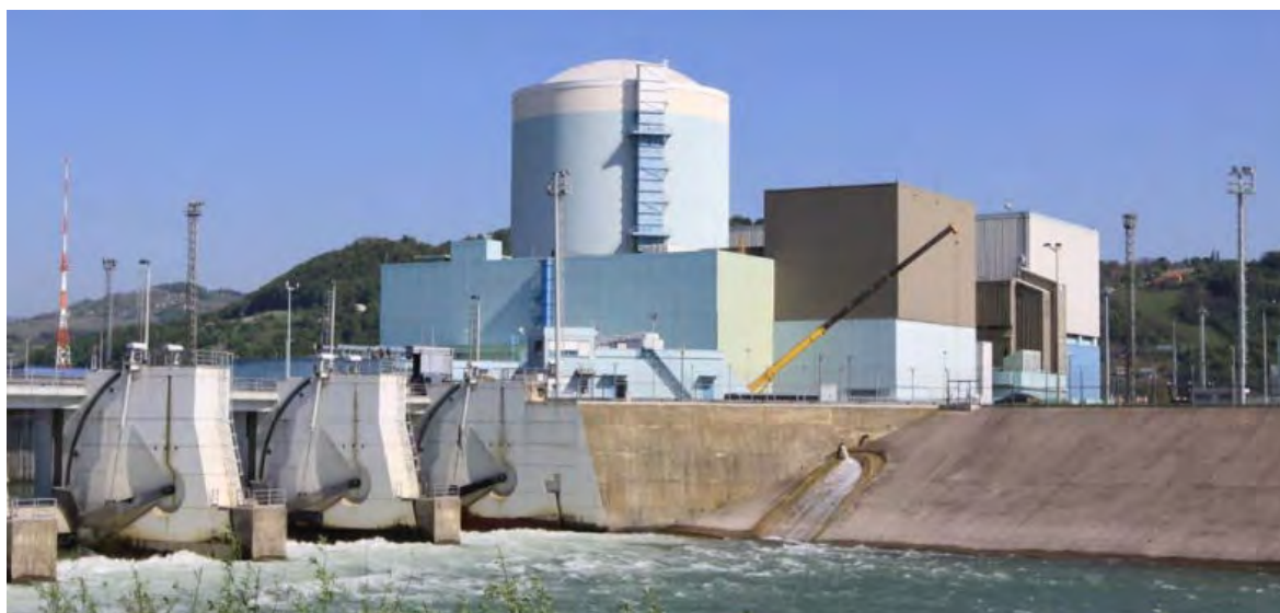
Slovenian-Croatian Krško Nuclear Power Plant. Photo by GEN Group.
