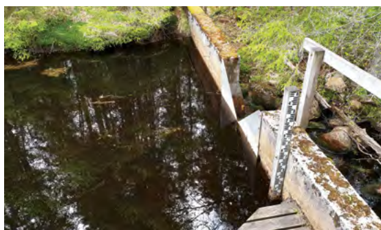
Measuring weir for flow measurement in the outlet section of the Birkenes research catchment in Norway. Photo by J. Čuřík.
