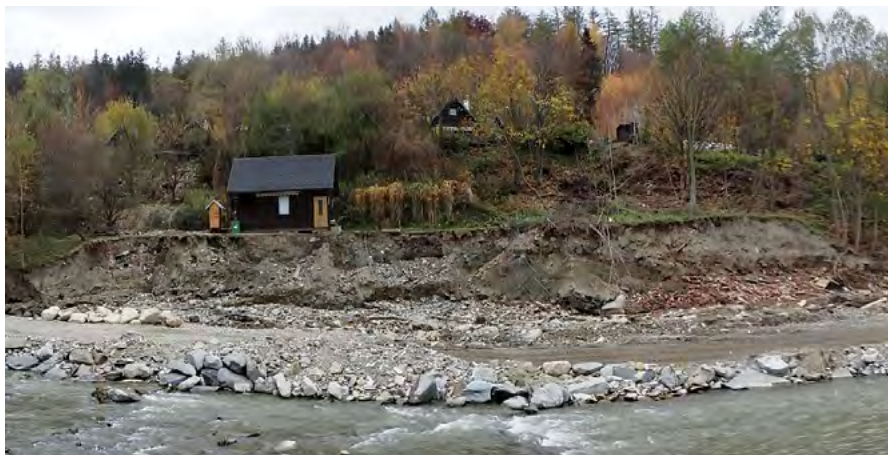
Washed-away accumulation part of the landslide in Vrbno pod Pradědem after the floods in September 2024. Photo by O. Krejčí.
