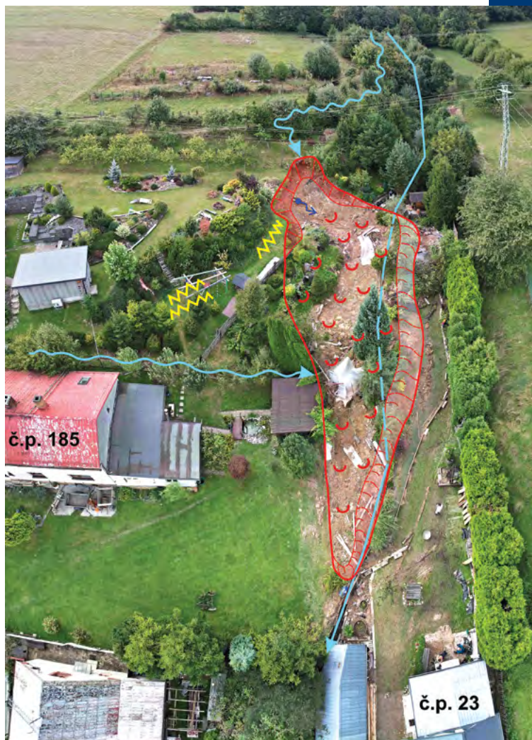
Schematic situation of the unstable slope at property No. 23 on the bank of the Myslíkovský stream in the cadastral area of Myslík, with a view to the west on the background of an aerial photograph taken by the CGS on September 19, 2024. Photo by J. Malík, September 2024.
