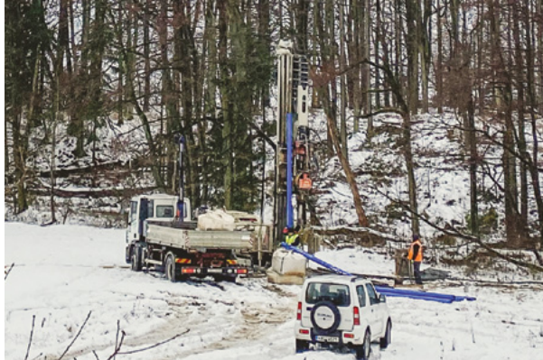
▲ Martínkov well drilled to a depth of 50 m during the “Groundwater in Crystalline Rocks” project. Photo by R. Hadacz.
