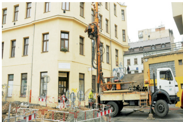
▲ Drilling of an engineering geology borehole with a depth of up to 30 m on the sidewalk on Anenská Street in Brno to determine the depth of the landslide's rupture surface. Photo by O. Krejčí.
