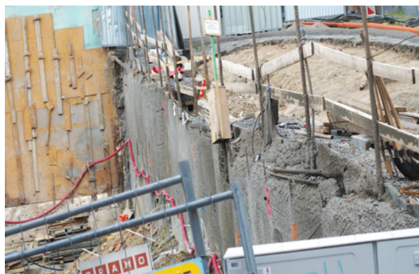
▲ Main scarp of an old landslide in a construction pit at the Leitnerova and Kopečná street intersection in Brno. Photo by O. Krejčí.
