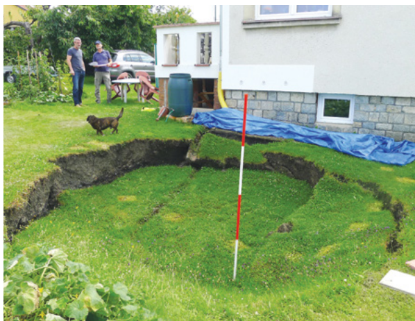
▲ Collapse of an old shaft in the garden of residential home in Rudolfov, České Budějovice district. View from W. Documented in the Mine Working Impacts Inventory.
