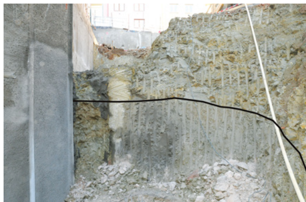
▲ Reactivation of an old landslide during a construction pit excavation at the Leitnerova and Kopečná street intersection in the built-up part of the city centre of Brno. Photo by O. Krejčí.
