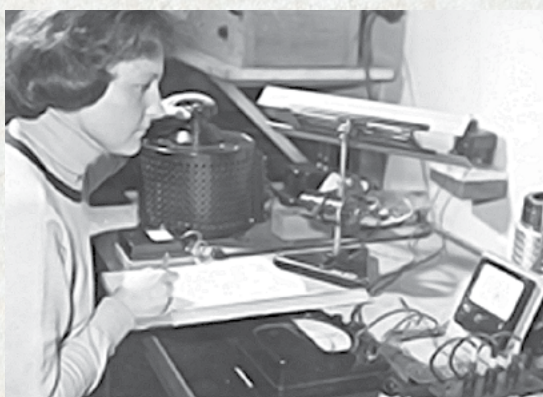
▲ DTA apparatus for identifying clay minerals. Photo by J. Bárta, 1960.
