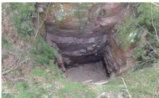
▲ A collapse of a ventilation shaft from the 4 th sinking near the former Mine 2 (Schacht II) at the Sn deposit between Jelení and Rolava was dealt with during the Mine Working Impacts Inventory project. Photo by Pavel Šír.
