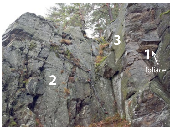
▲ View from the bottom of a rock formation in Řetenice u Stach showing three main systems of discontinuities. The overall loose rock formation and the self-help retaining rope system are clearly visible. Photo by J. Novotný.
