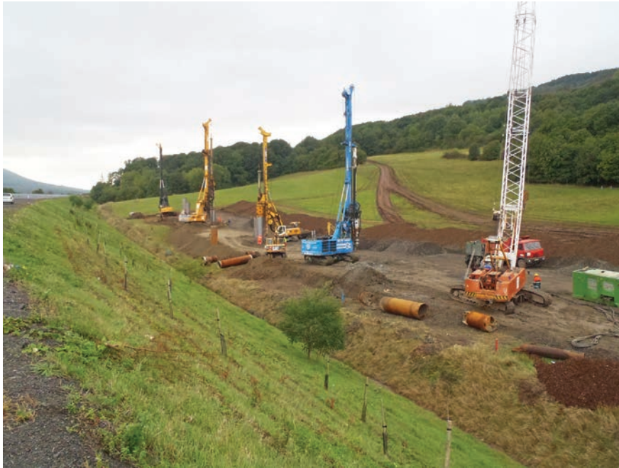
D8 motorway (km 57,400). Construction of an underground gravel wall along an earthwork with the aid of piles driven to a depth of 16 m. Photo by P. Kycl.
