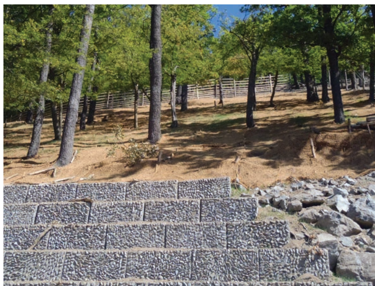
Remediation of steep erosion slopes on the left bank of the Klíčava Reservoir in the Lány Game Preserve.
