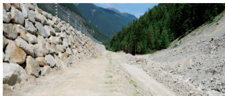
Interception area behind the retaining wall separating the road from the rock landslide at Umhausen in the Tyrol (photo by O. Krejčí).
