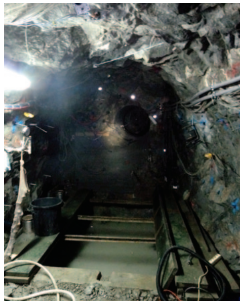
The location of the experimental site and instrumentation in the Josef Gallery near Mokrsko used for the project Research on thermally loaded rocks . The picture shows the site before isolation of the wide-diameter heating borehole and surrounding monitoring boreholes.
