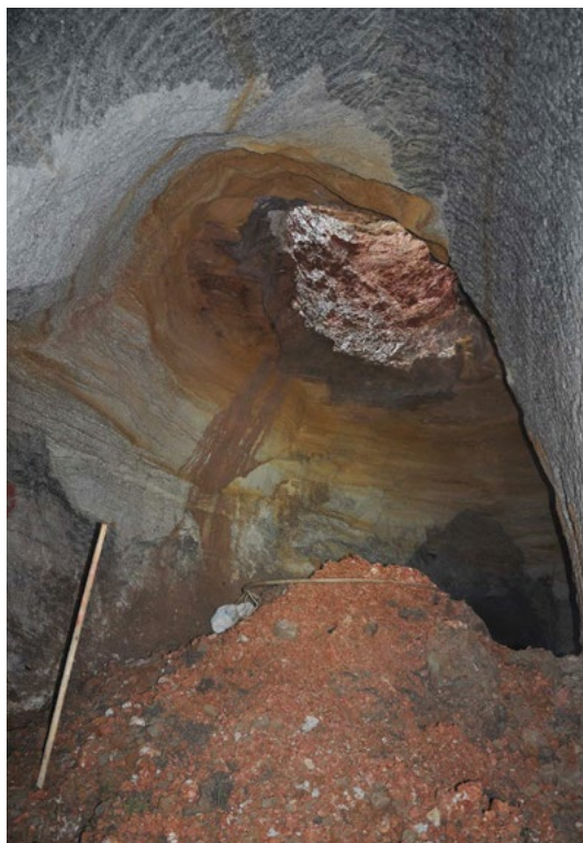
A sinkhole in a former kaolin mine in Orty near Hosín, České Budějovice district. Documented in the Mine Working Impacts Inventory.
