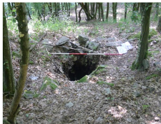
A sinkhole in the lower adit under Dušno in the locality of Hradištko pod Medníkem, Prague-West district. Documented in the Mine Working Impacts Inventory.
