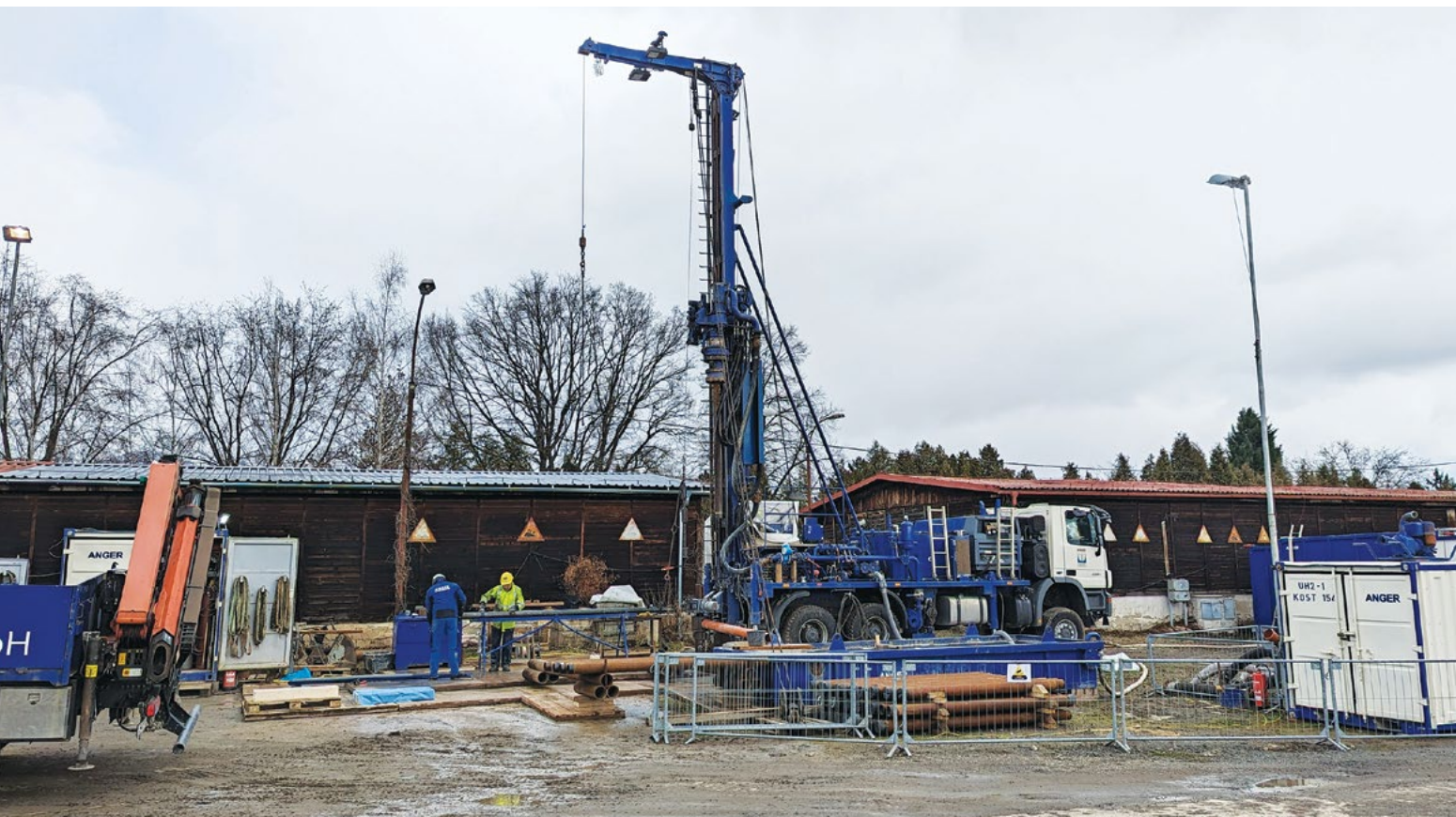
Drilling of a 500 m deep borehole at Litoměřice. This is the first exploratory borehole of the prospective BTES repository. Photo by J. Holeček.
