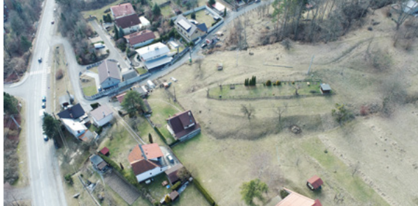
► Monitoring of slope deformations from 1997 with a CGS drone. Slope deformation 25-32-05/82 Vsetín – House of Prayer. Photo by J. Nečas.
